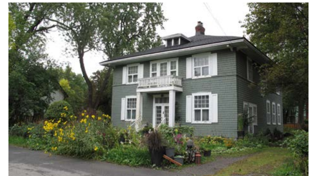
Bowling Green Avenue single-family home Source: Provencher_Roy, 2019
