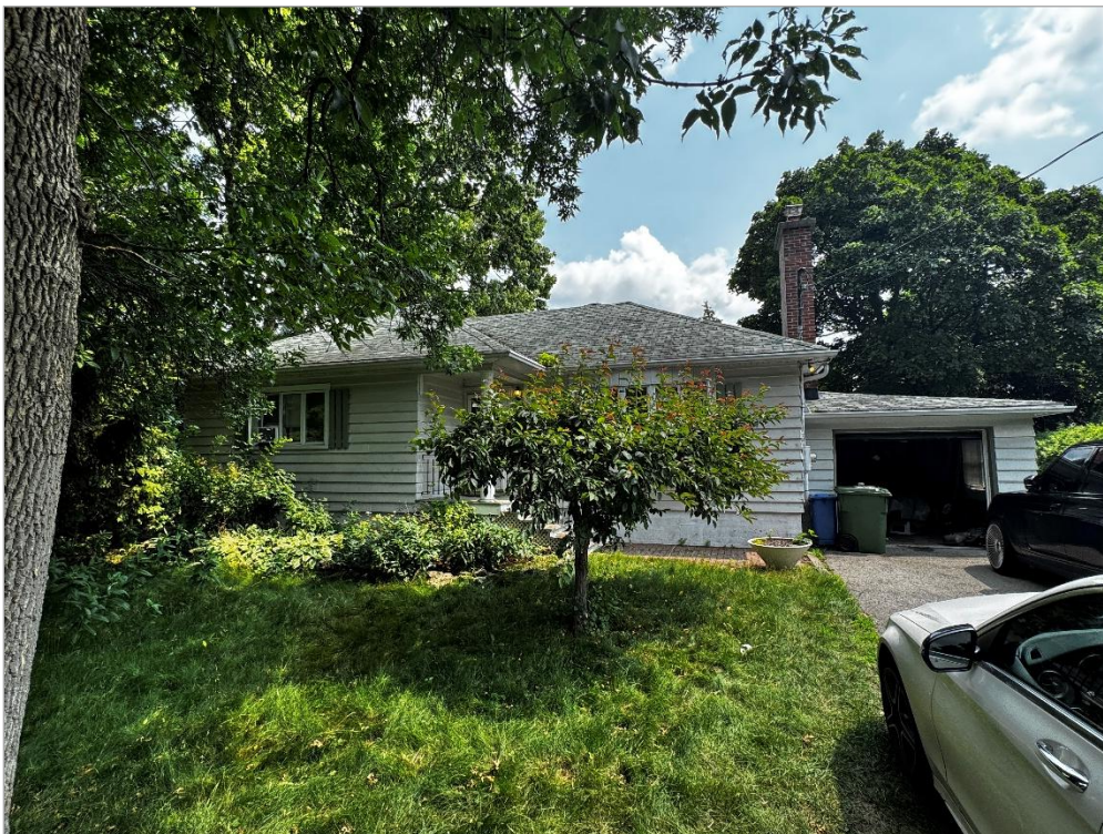
Front view of the building
