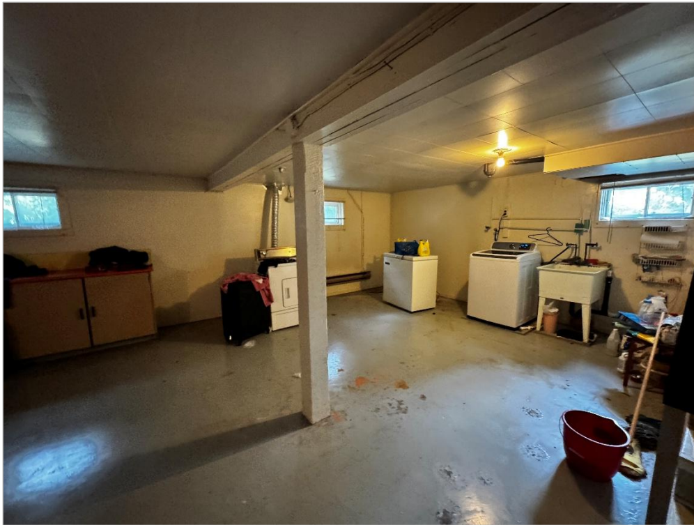
Basement and laundry area
