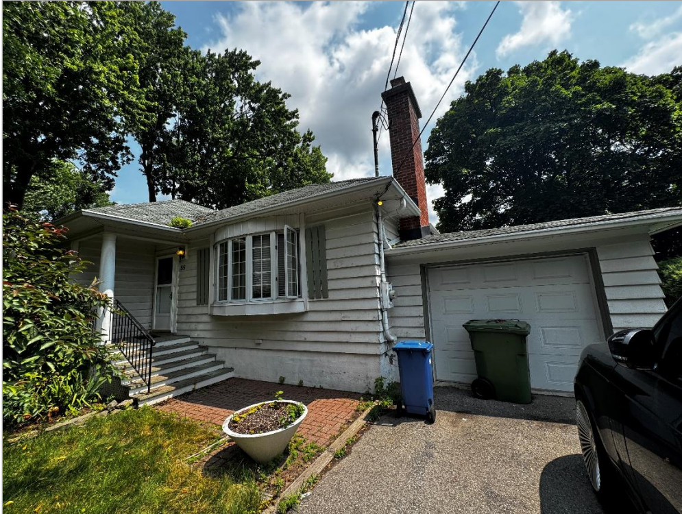
Front view of the building
