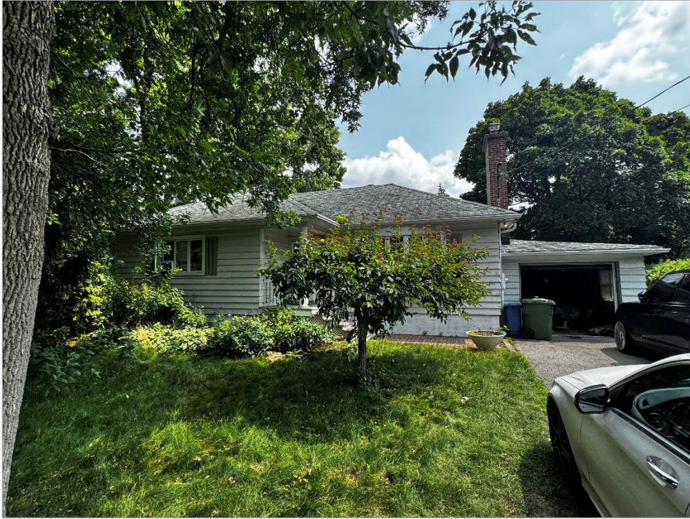
Front view of the building
