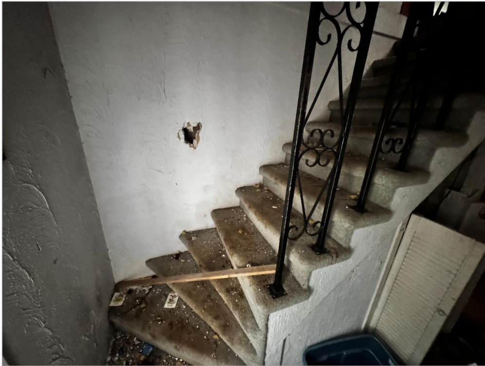
Staircase to the upper floor
