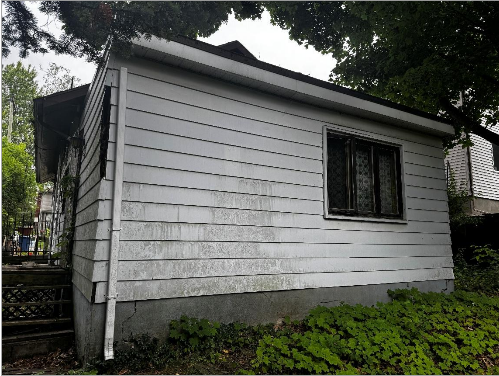
Rear view of the building
