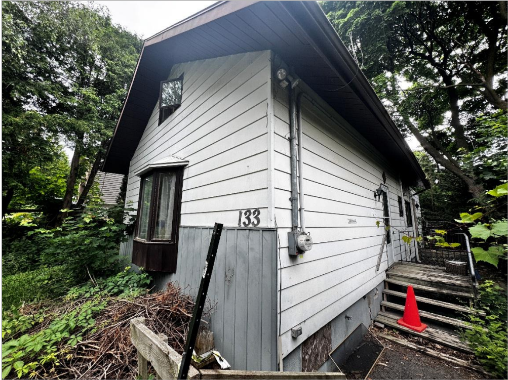
Right view of the building
