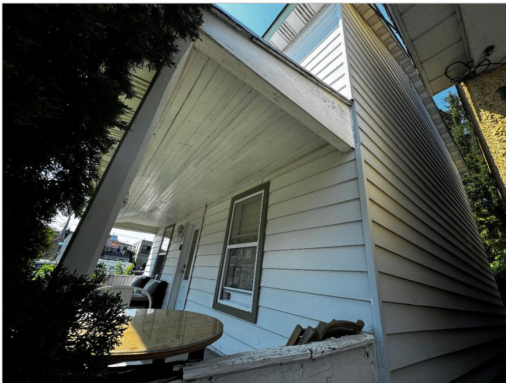
Right elevation of the building
