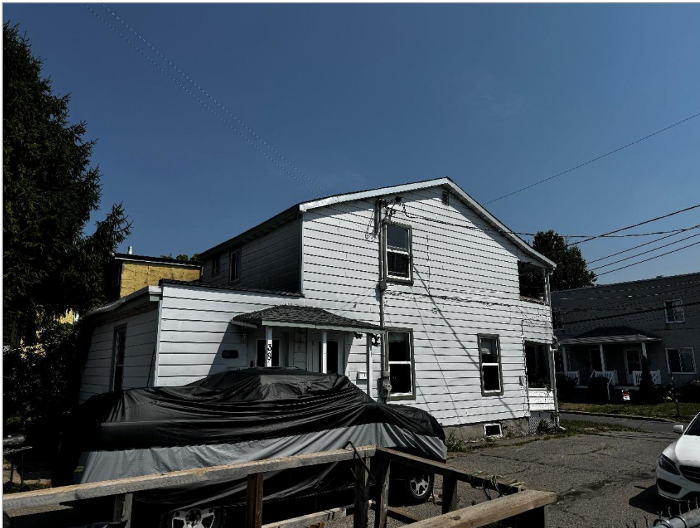
Left elevation of the building
