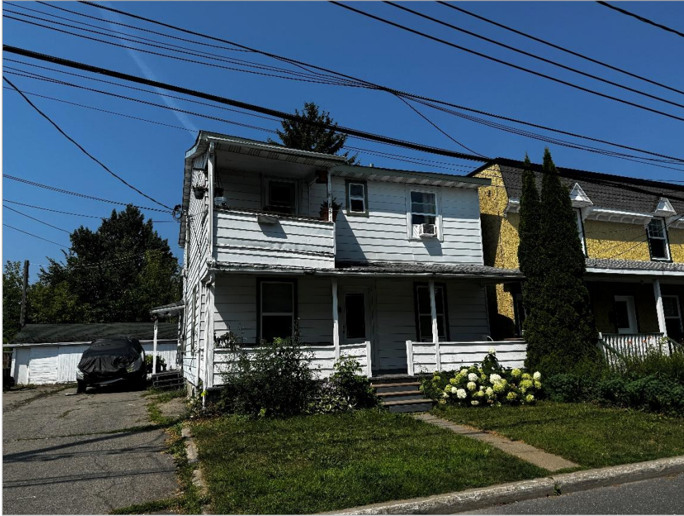
Front view of the building
