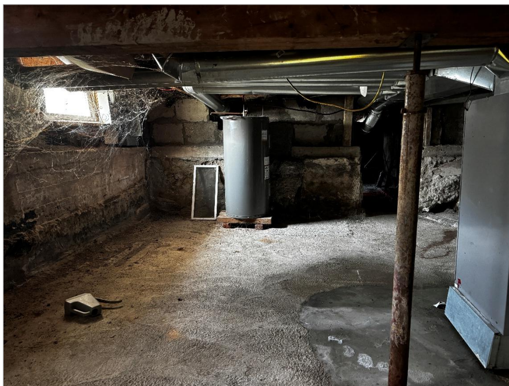
Service basement (accessible through the unit 38, Saint-Joachim)
