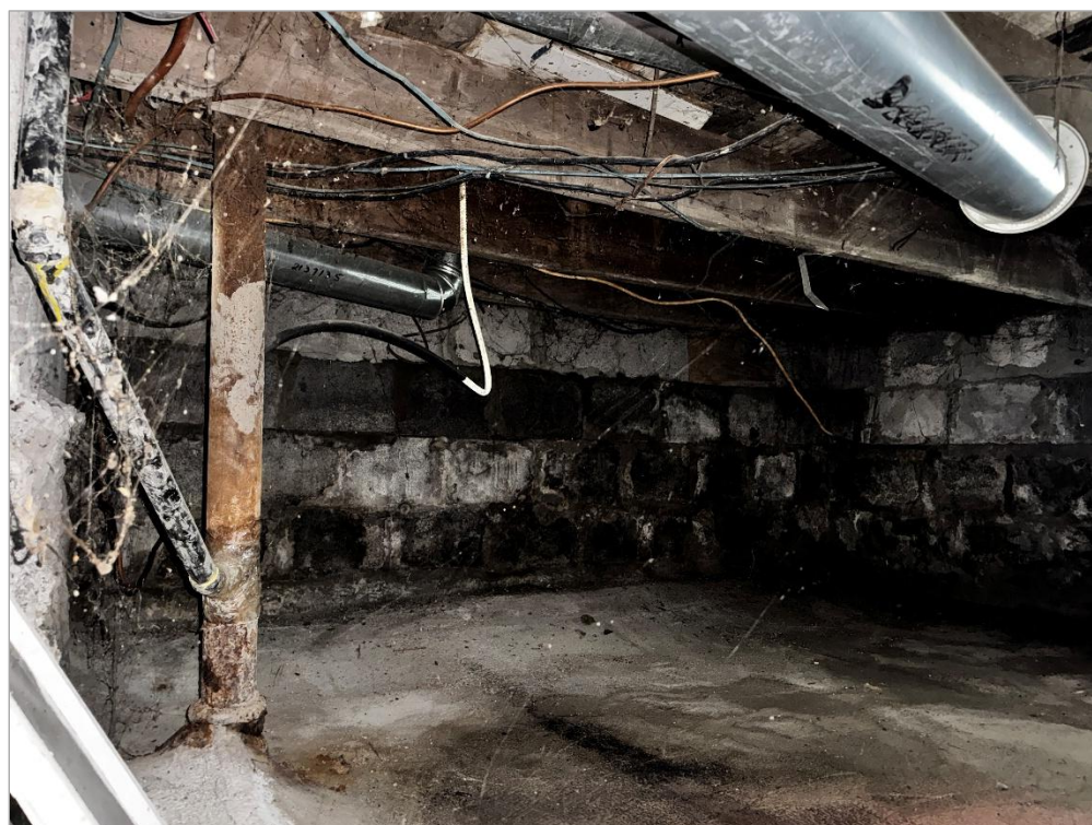
Service basement (accessible through the unit 38, Saint-Joachim)
