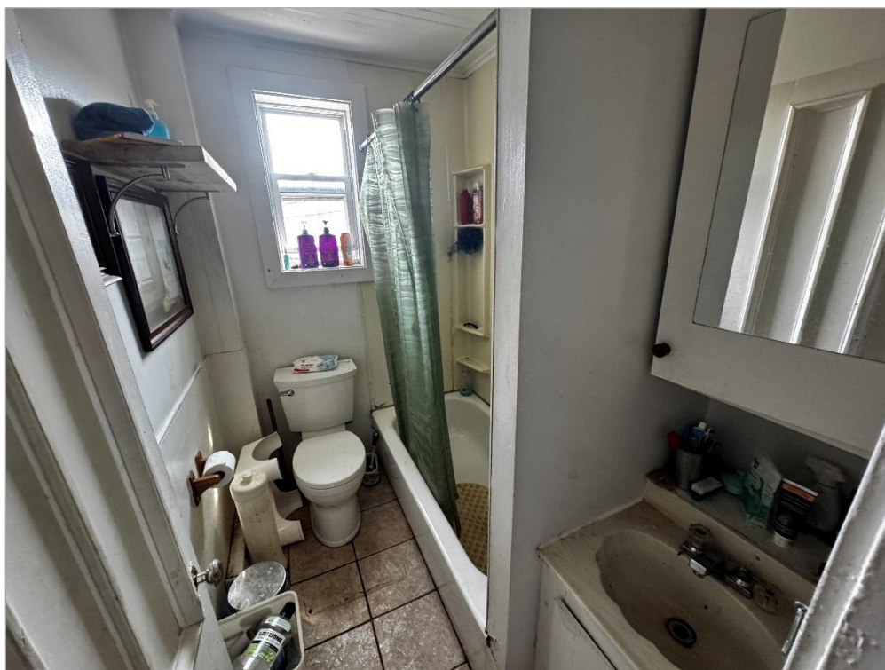
Bathroom on the second floor (unit 38A, Saint-Joachim)
