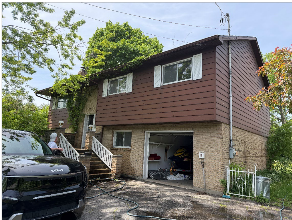
Front view of the building
