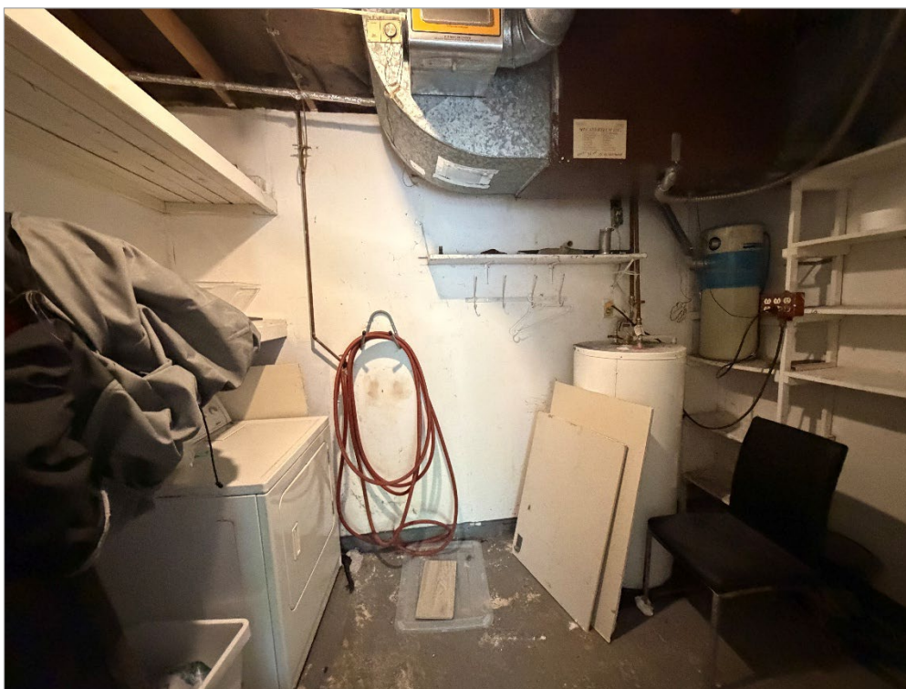
Laundry and mechanical room (ground FLOOR)
