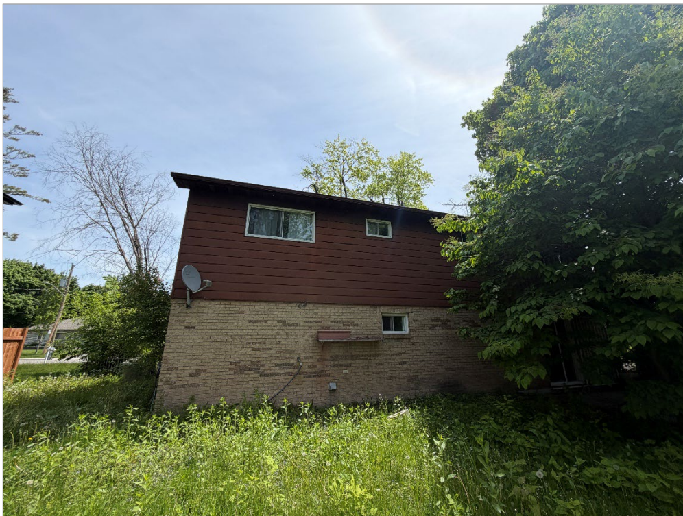
Rear view of the building
