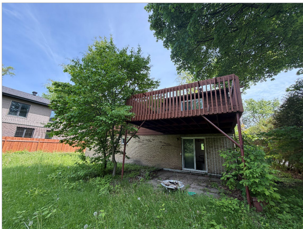
Rear view of the building
