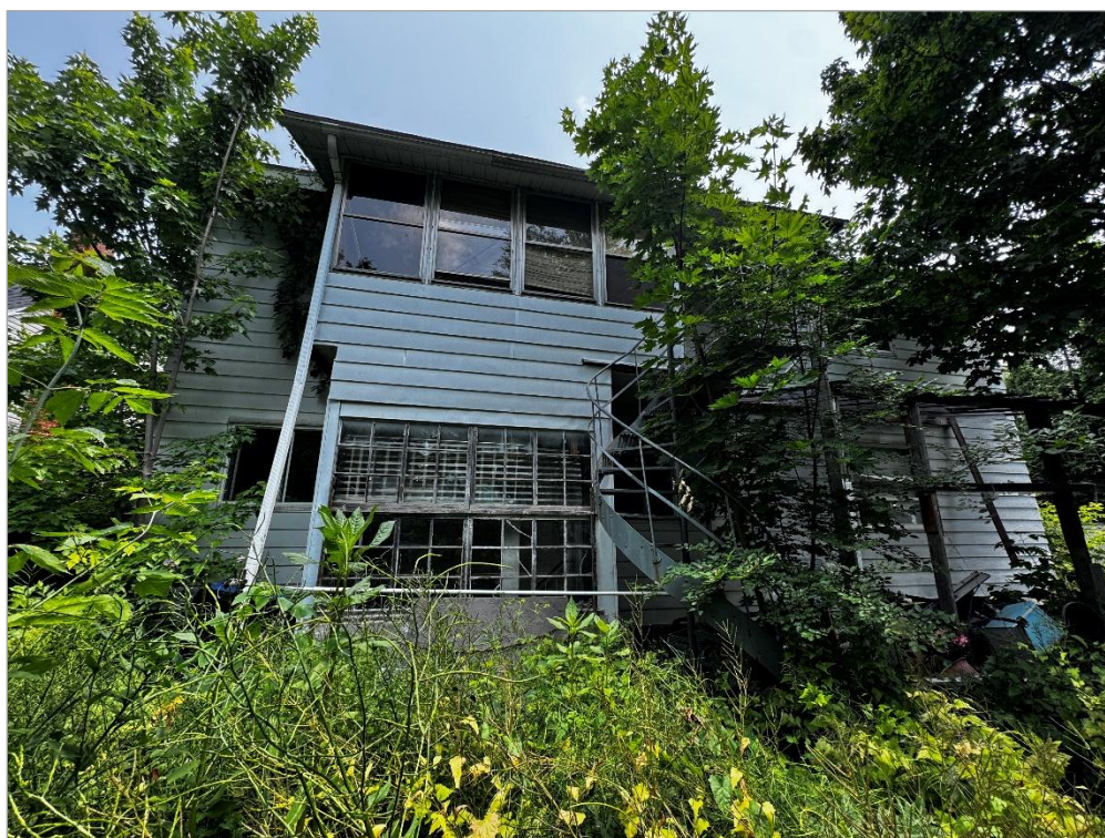
Rear view of the building
