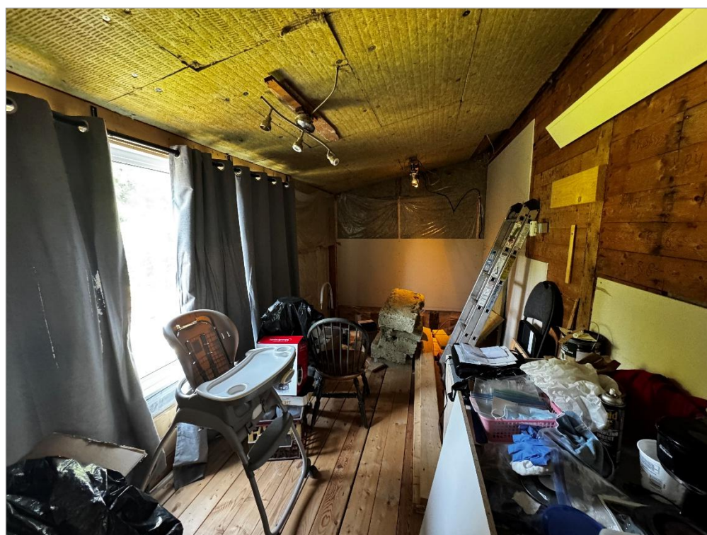
Dining room (currently under renovation).
