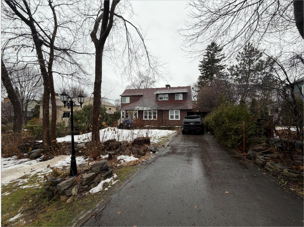
Front view of the building
