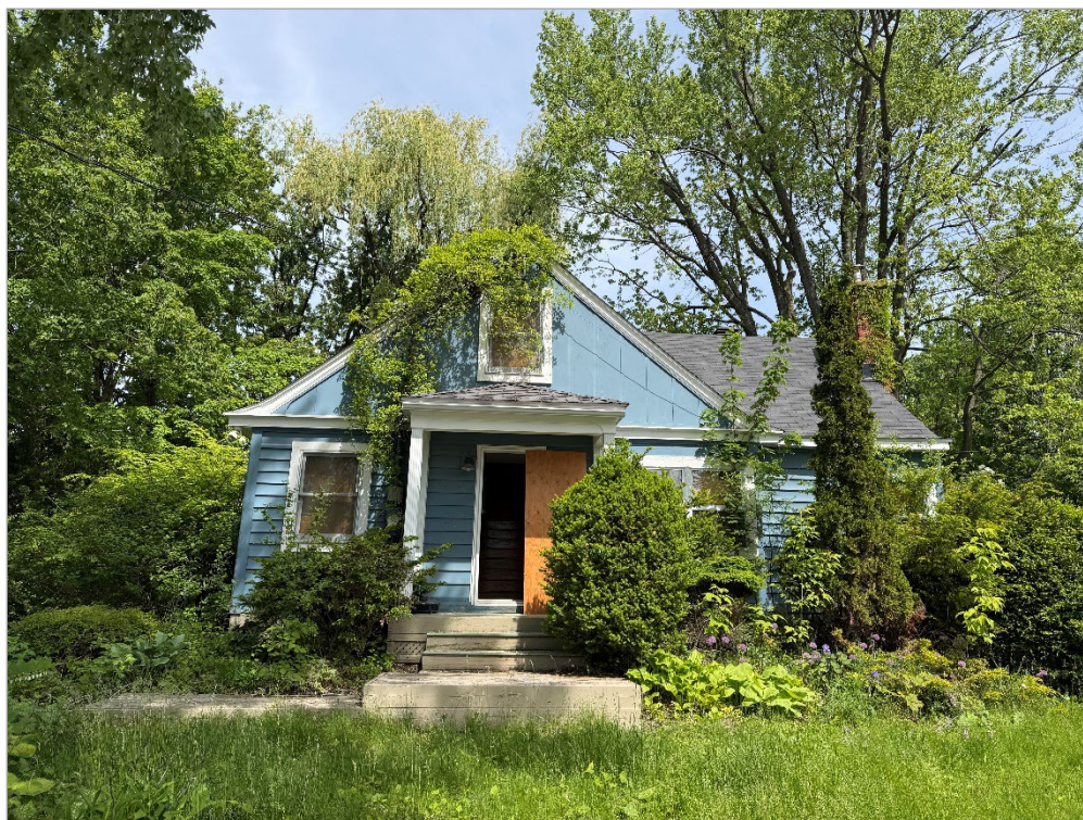
Front view of the building
