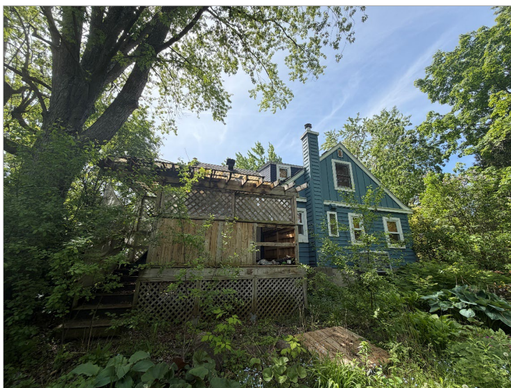
Rear view of the building
