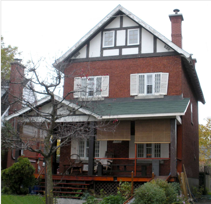
Example of an Arts & Crafts house that requires maintenance on the woodwork, repairs to trim that has deteriorated and replacement of most of the components of the front porch, all at the same time.
