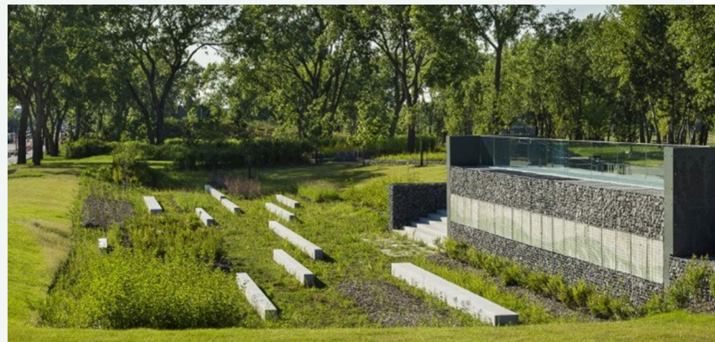
Example of successful integration of retention basins in Frédéric-Back Park (Saint-Michel district, Ville de Montréal).
