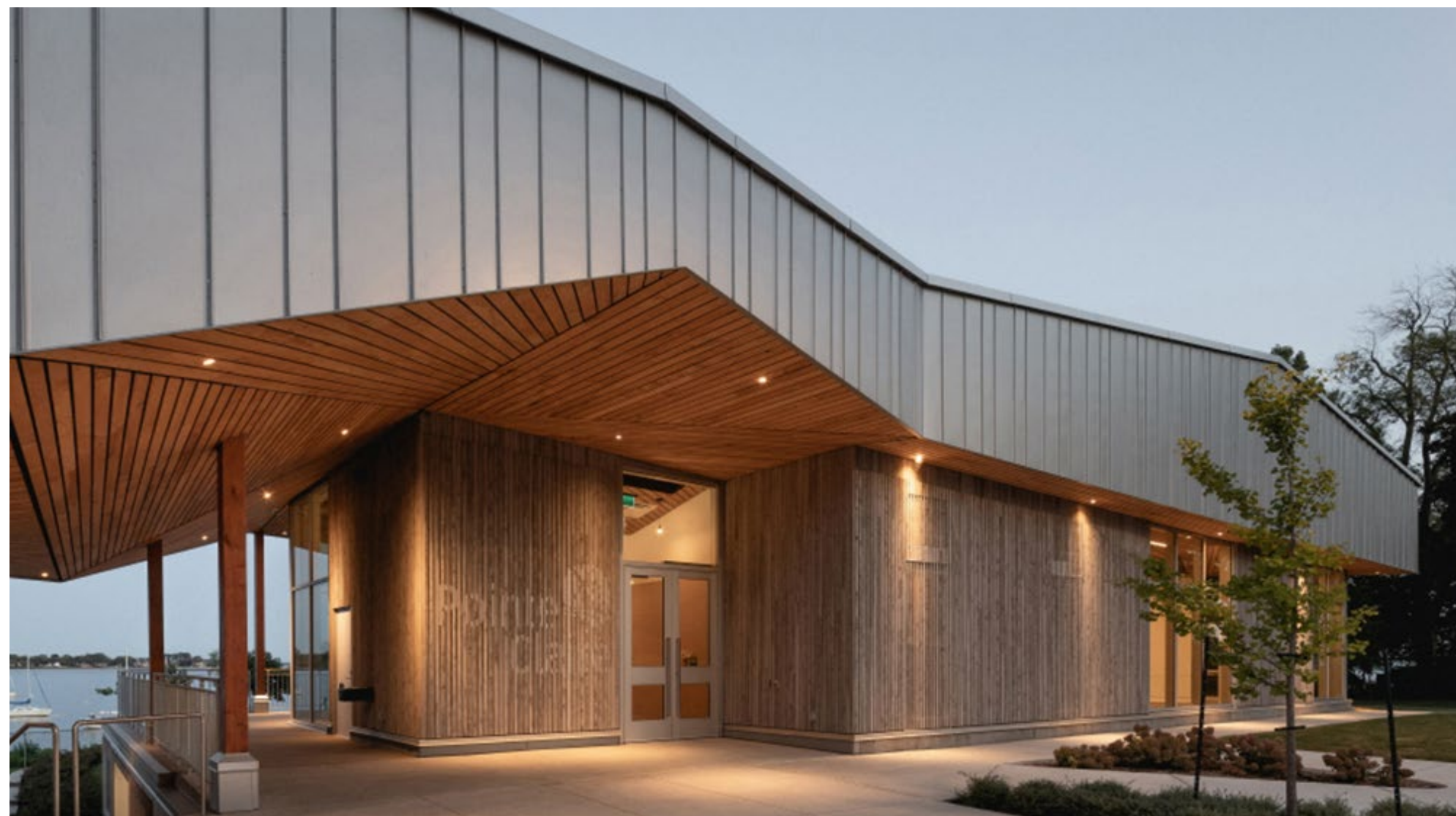
Baie-de-Valois chalet at Grande-Anse Park, City of Pointe-Claire
